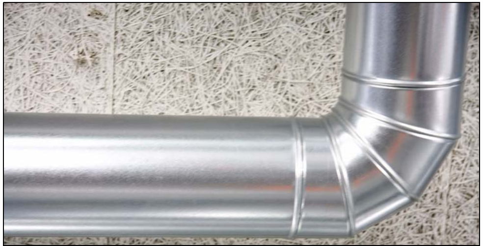
Installation of folded spiral-seams ducts
